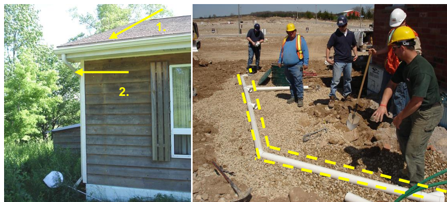
Figure 1-1. [LEFT] 1. Gutter and 2. Downspout; [RIGHT] Conveyance drainage piping for below-ground rainwater storage tank (prior to burial)
