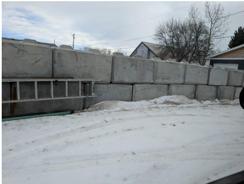
Figure 16 - Concrete fence in residential area
