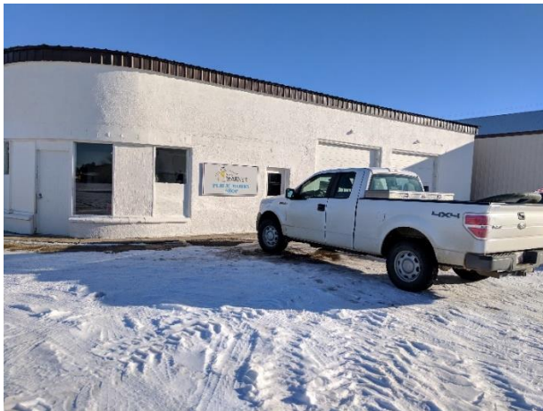
Figure 11 - Warner Public Works Shop
