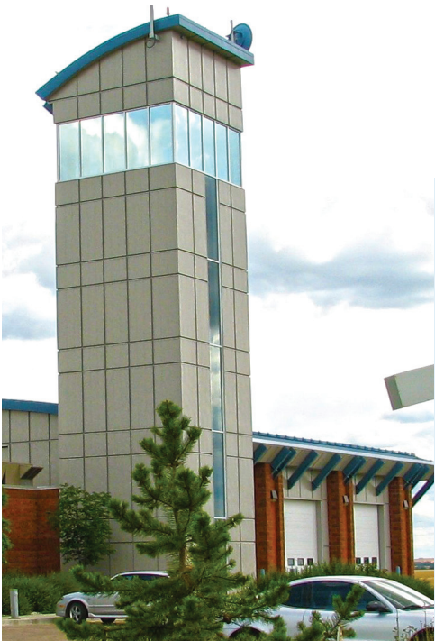
Station #4 Heartland Hall, Strathcona County
