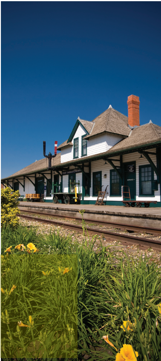
CN Station, Fort Saskatchewan
