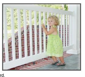
Horizontal members are not permitted between 140 mm (5  $\frac{1}{2}$ ") and 900mm (36") above the finished floor surface.
